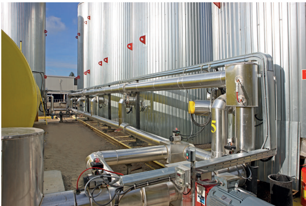
Electrically heated pipes in InNOVA 320 plant (Poland).
