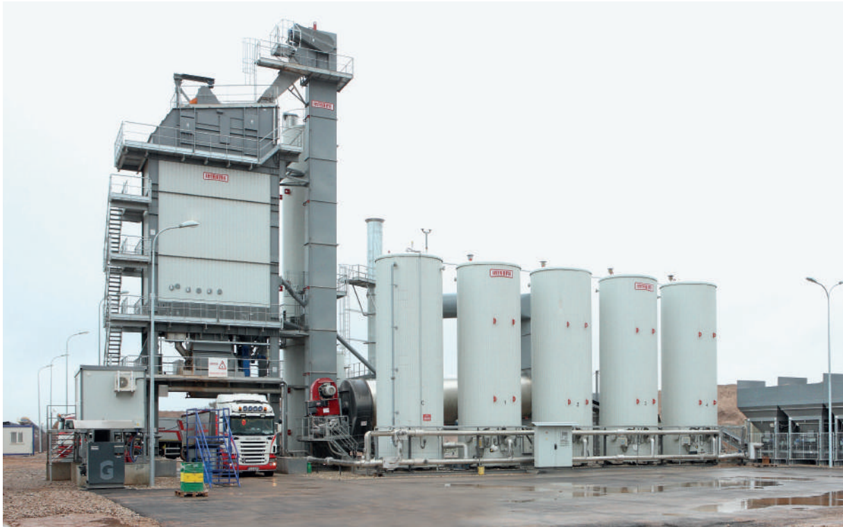
320 t/h asphalt plant (Poland). With InNOVA-G mixing tower. Equipped with 160 t capacity hot bins. Bitumen tanks electrically heated. Installed on metallic foundations. 4.500 kg mixer.
