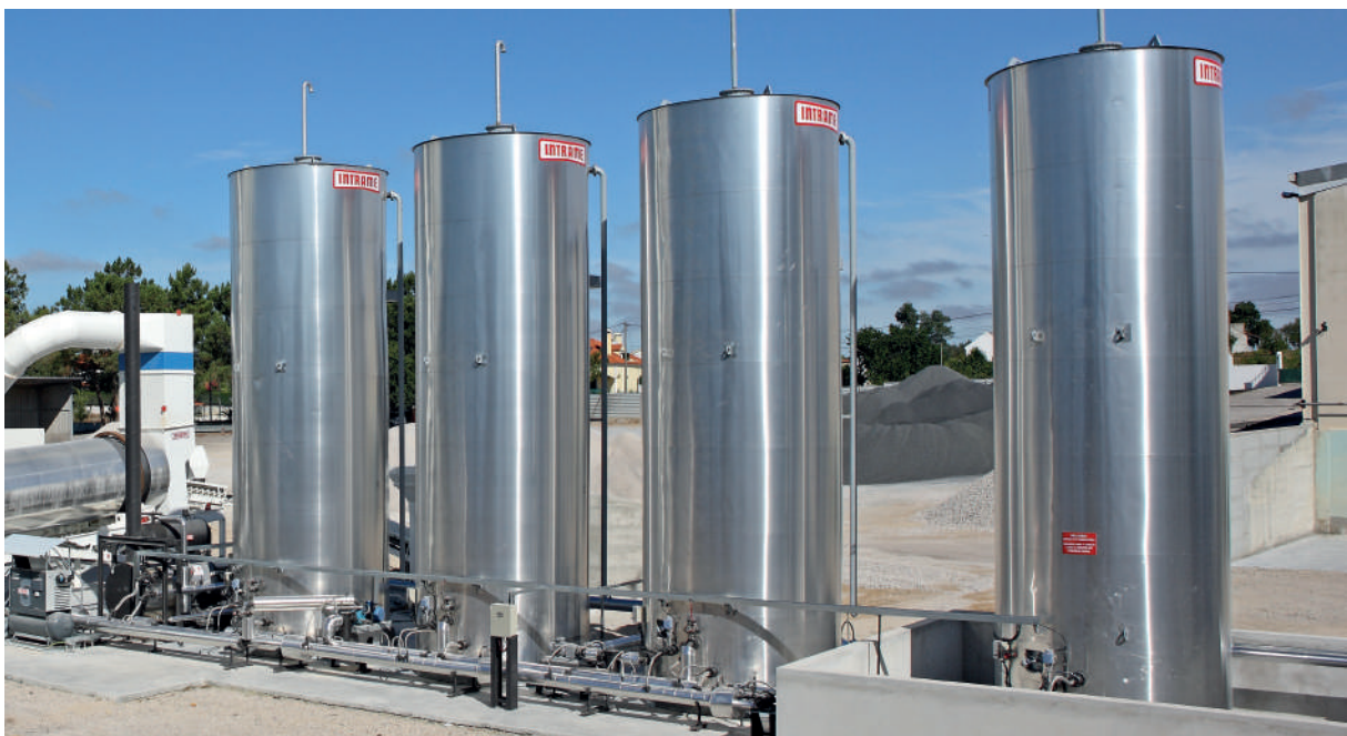
Vertical tanks heated by thermal oil.
